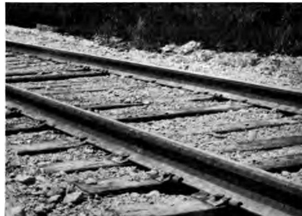
P. & M. Rail Anti-Creepers on Southern Pacific Company through Suisun Swamp, near Suisun, California
